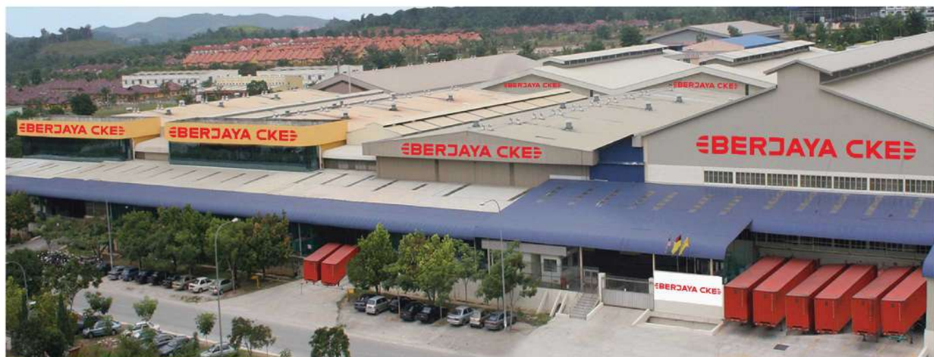
Manufacturing Plant In Negeri Sembilan, Malaysia
